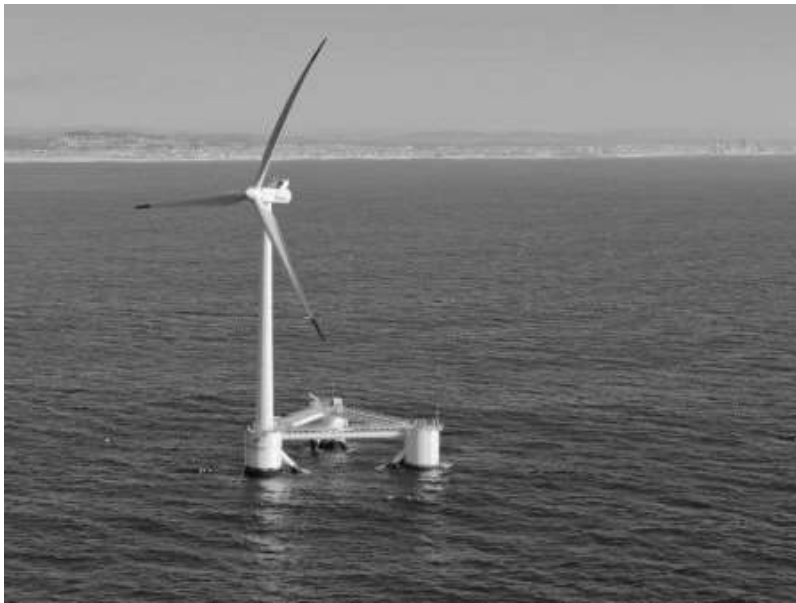
Figure 5. Floating WPP in Japan 23 km from Fukushima
