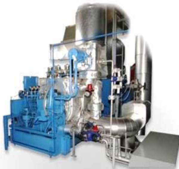
Figure 3. Mini cogeneration plant working with wood wastes
