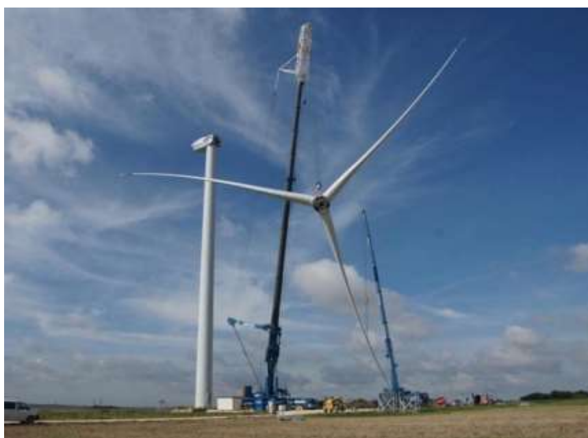
Figure 3. The process of installing a wind generator
