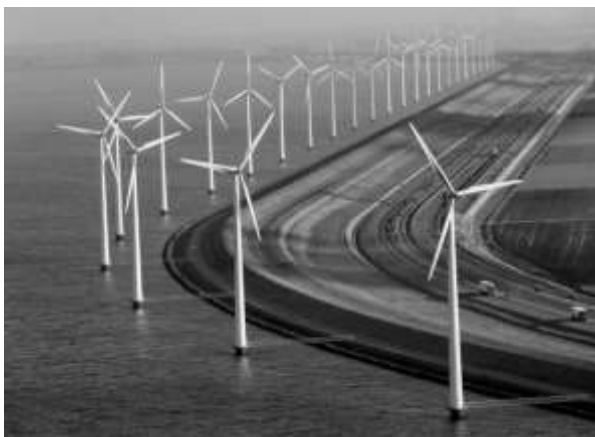
Figure 2. Novoazovskaya onshore WPP
