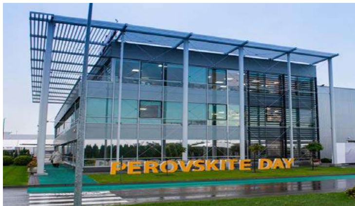
Figure 1. Building with photovoltaic blinds [1]
