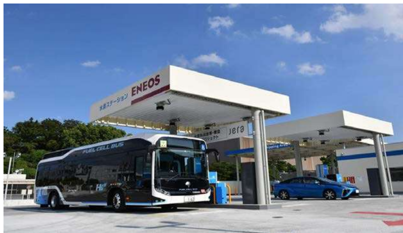
Figure 3. Hydrogen Vehicle Refueling Station in Japan [5]
