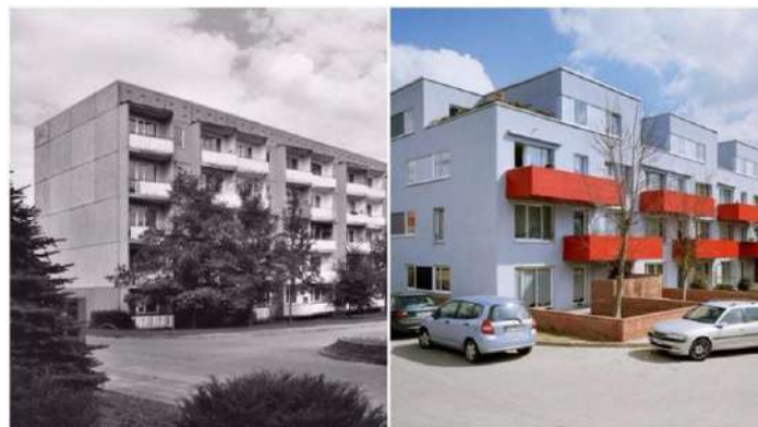
Figure 13. The renovated panel building. Leinefelde-Worbis, Germany
