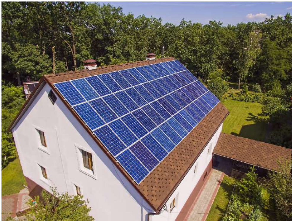
Figure 2. Use of solar panels on the roof of the house
